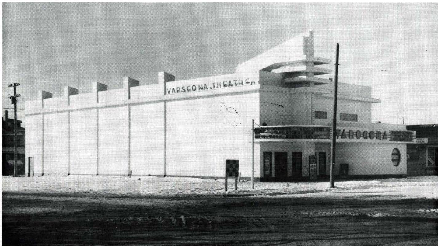
Both the Varscona Theatre and the Eaton's department store were built in 1939 and demolished in 1987.
