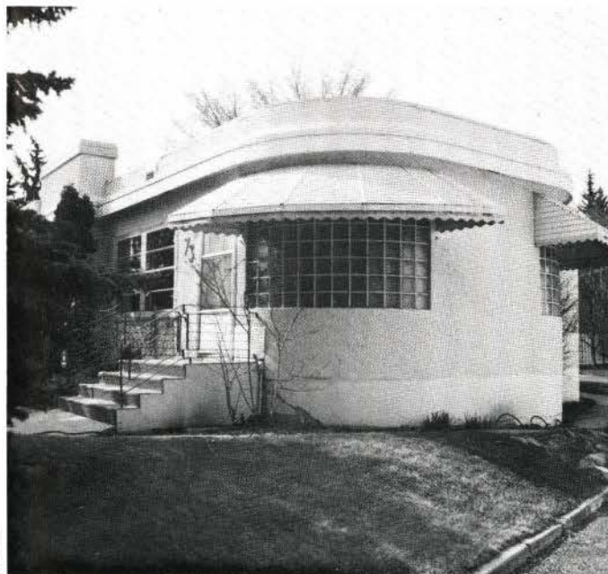
73 Ravine Drive, one of Edmonton's finest examples of residential Moderne.
