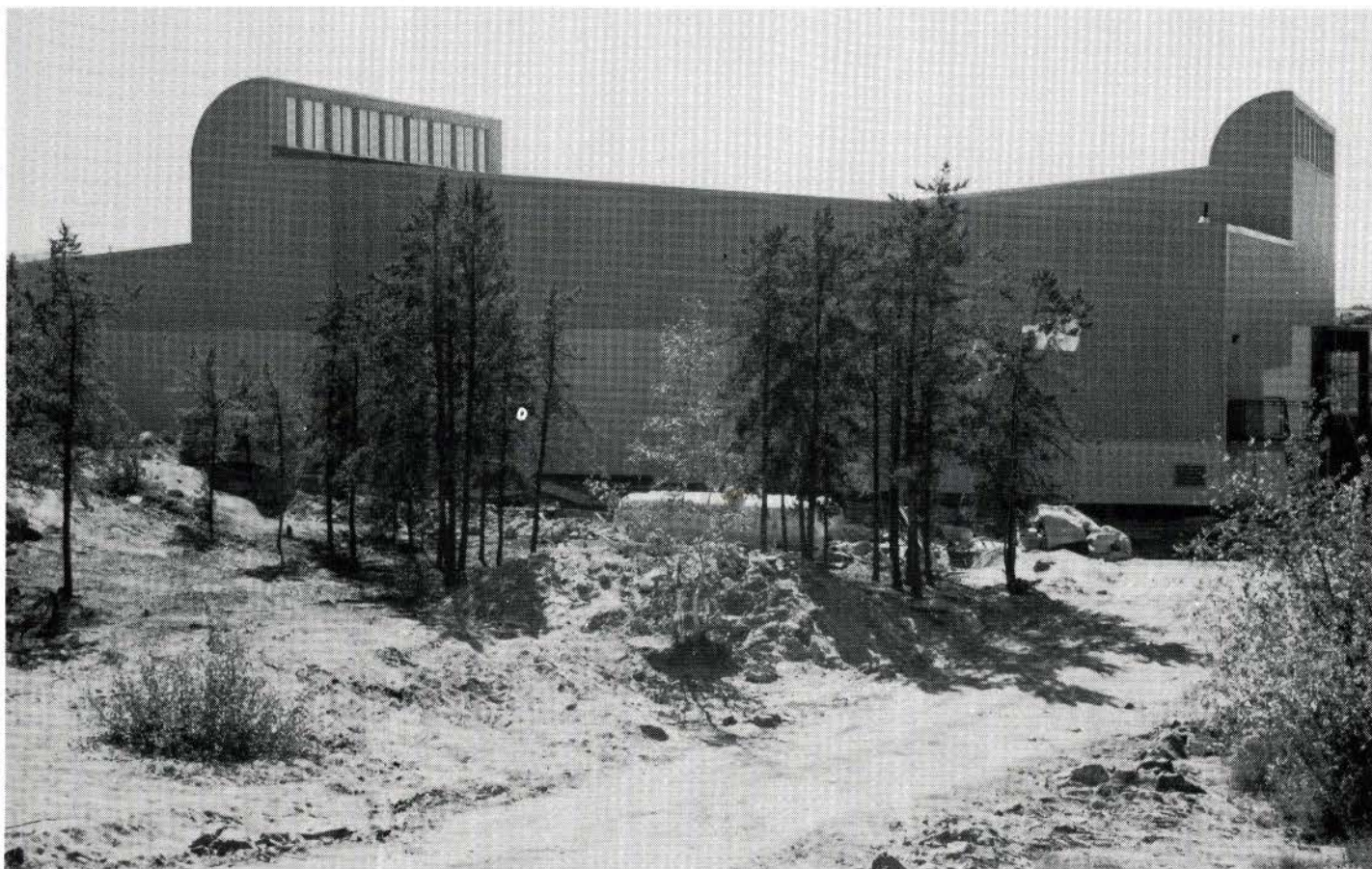
New recreational complex for the City of Yellowknife. Facility includes a wave pool and 8 sheet curling rink.
