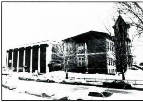
Figure 19 (right). Perspective of the front and side facades of the Édifice Federal, Valleyfield, Quebec, circa 1965. (06 ARC 025N)
