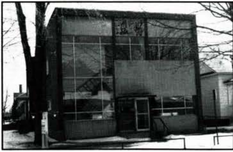
Figure 2. View of the principal facade of the Brassard Medical Centre, Valleyfield, Quebec. David Rose, photographer. (06 ARC 042N)
