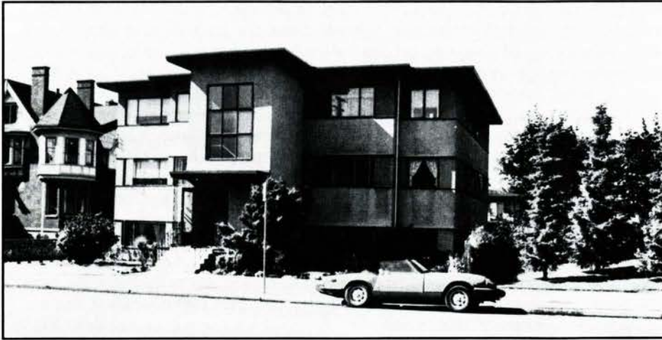
Figure 3. An apartment house on Fort Street in Victoria, designed by Marjorie Hill in 1952. (University of Toronto Archives)
