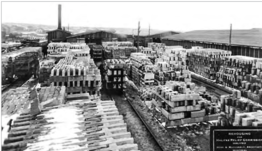
FIG. 12. CANADIAN HYDROSTONE PLANT, EASTERN PASSAGE, JANUARY 1919. THE PLANT WAS BUILT IN ORDER TO ACCELERATE HOUSE RECONSTRUCTION. | NOVA SCOTIA ARCHIVES AND RECORDS MANAGEMENT, WILLIAM SMITH COLLECTION, ACCESSION NO. 1991-325, NEGATIVE NO. N-7050.
