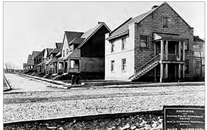
FIG. 14. NEWLY BUILT HYDROSTONE HOUSES DESIGNED BY ROSS AND MACDONALD. THIS STRIP OF HOUSES IS LOCATED ON THE NORTH SIDE OF SEBASTIAN PLACE, WEST OF GOTTINGEN STREET. | GAUVIN AND GENTZEL, MARCH 24, 1921. NOVA SCOTIA ARCHIVES AND RECORDS MANAGEMENT, WILLIAM SMITH COLLECTION, ACCESSION NO. 1991-325, NEGATIVE NO. N-7015.
