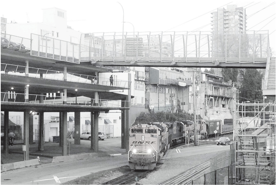
View of parking structure from waterfront park
