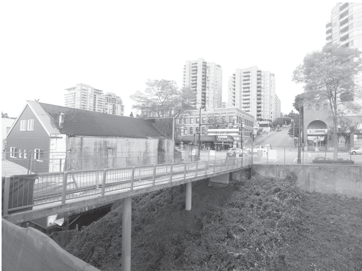
Steep grade change at the terminus of 4th St.
