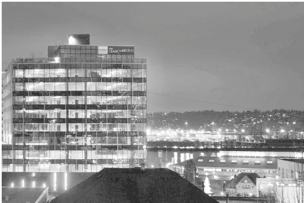
Completed in 2014, New Westminster's Anvil Centre remains unleased
