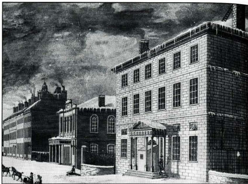
Figure 3. Detail of a view of St. James Street, Montreal, by Robert A. Sproule (1799-1845), engraved by William S. Leney (1769-1831), and published by A. Bourne, Montreal, 1830. On the right is the first office of the Bank of Montreal (Andrew White, architect, 1818-19). Beside it is the Wesleyan Methodist Chapel designed by John Try in 1820. (National Archives of Canada, C-16492)
