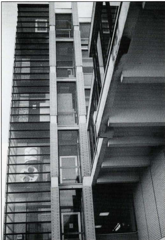
Figure 9. Hebb Building, University of British Columbia, Vancouver; Thompson Berwick Pratt & Partners, architects, 1962-63. (M. McMordie, 1988)
