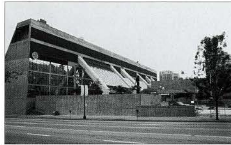
Fig. 17. Thompson Berwick Pratt and Partners, CBC Building, 1973-75, Vancouver. (photo L. Noppen)
