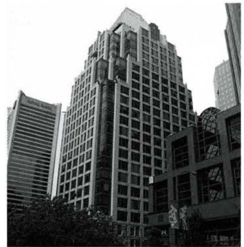
Fig. 14. Paul Merrick, Cathedral Place, 1989-91, Vancouver. (photo L. Noppen)
