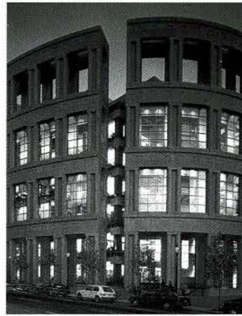
Fig. 17. Southwest elevation: Robson and Homer Streets (photo T. Hursley). (Moshe Safdie Archive, CAC, McGill University Libraries)
