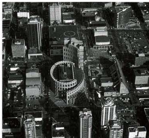
Fig. 19. View of southeast corner: Robson and Hamilton Streets. (Moshe Safdie Archive, CAC, McGill University Libraries)
