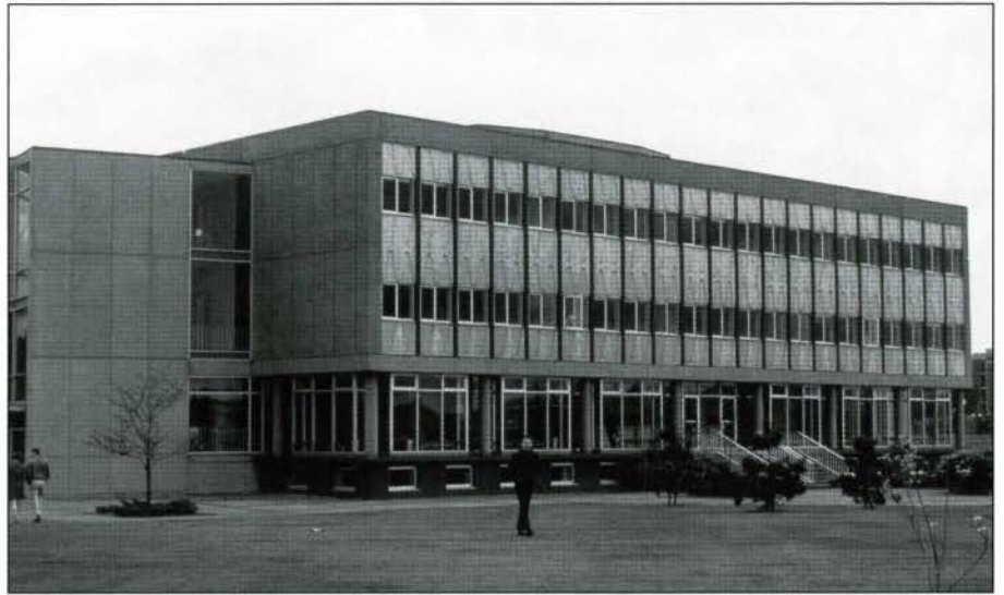
Fig. 6. Wade Stockdill & Armour. Clearihue Building, University of Victoria, 1962. (photo Chris Gower)
