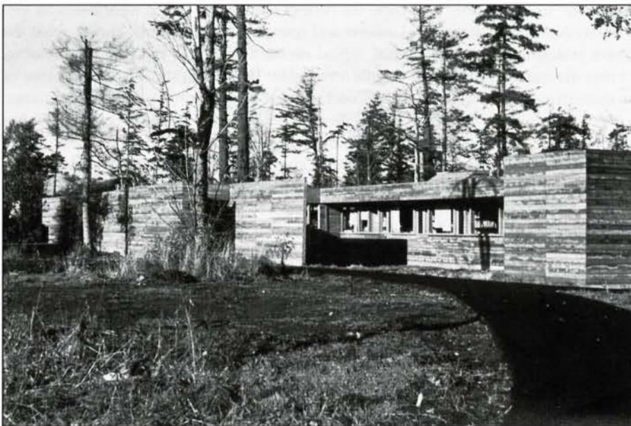
Fig. 5. Barry V. Downs. Sedgewick Building, University of Victoria, 1968-1969. (University of Victoria, History in Art department slide collection)
