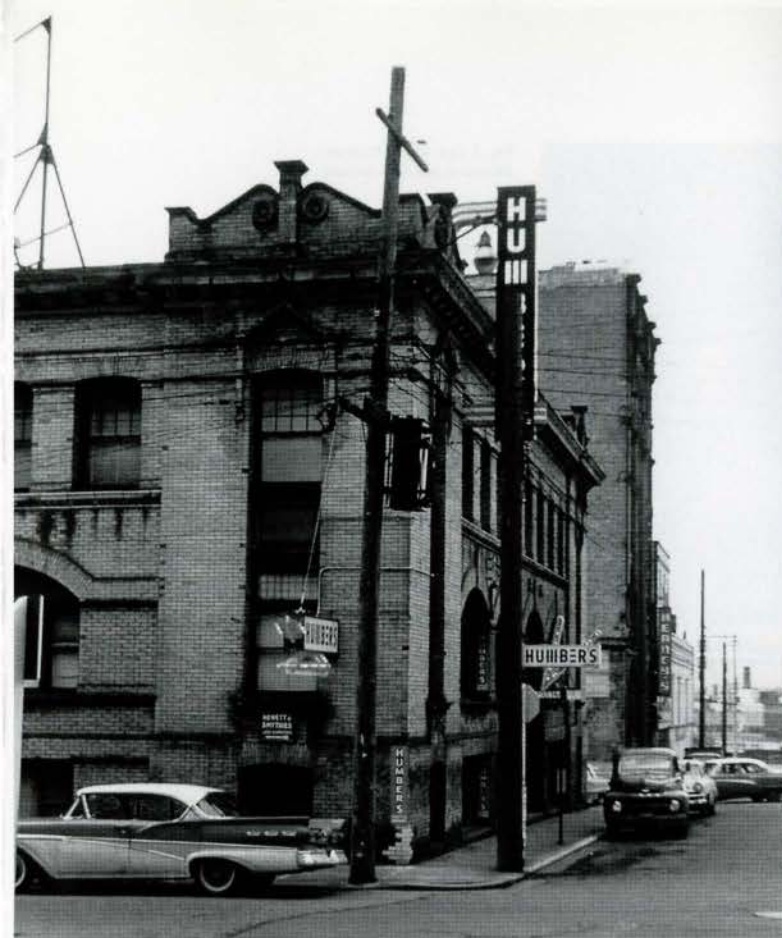
Fig. 1. Corner of Bastion Square (right) and Langley Street (left), Victoria, before restoration, ca 1959. Nearest building is Law Chambers, architect Francis M. Rattenbury, 1899. (Photo by Peter Cotton. Collection of Chris Gower)
