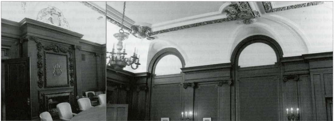
FIG. 19 a-b. DETAILS OF THE ORIGINAL WOOD FITTINGS IN THE CABINET ROOM, INCLUDING THE FIREPLACE, THE WOODWORK —PILASTERS, ARCHES AND PANELING— GILDED PLASTER WORK, AND AN ORIGINAL MAXWELL CLOCK CASE. | R. GOODSPEED, 2004
