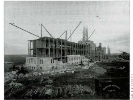
FIG. 28. LEGISLATIVE BUILDING UNDER CONSTRUCTION, IN 1910.
