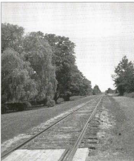
FIG. 18. RAIL TRACK, SOUTHERN BOUNDARY | WAYDE BROWN, 2006
