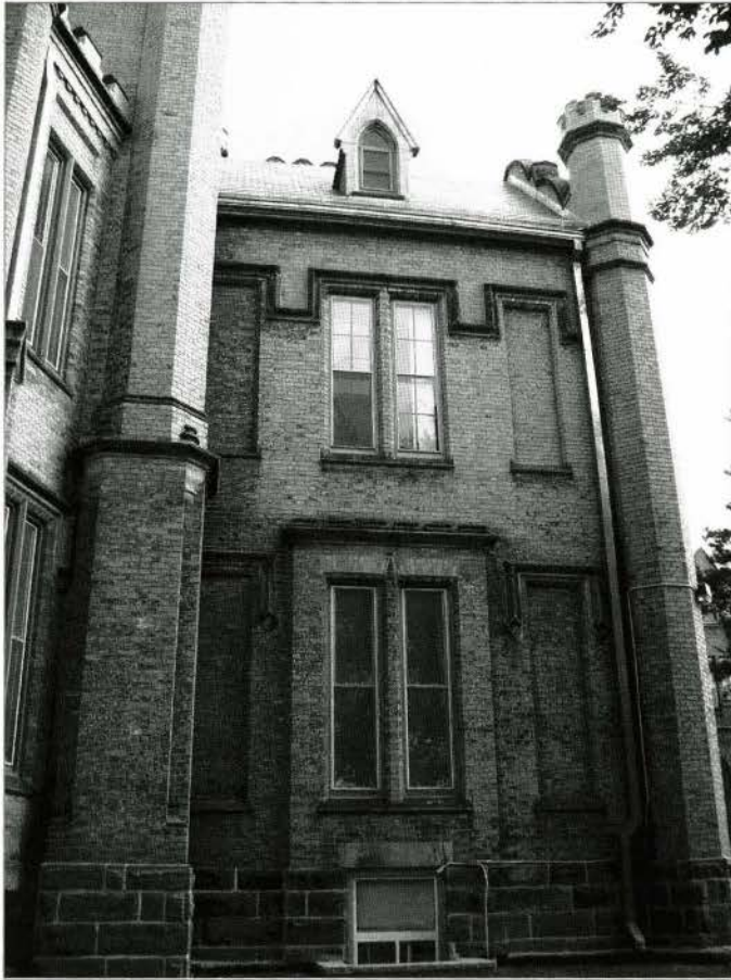
FIG. 4. RIGHT BAY OF FAÇADE. | PHOTO: JESSICA MACE.
