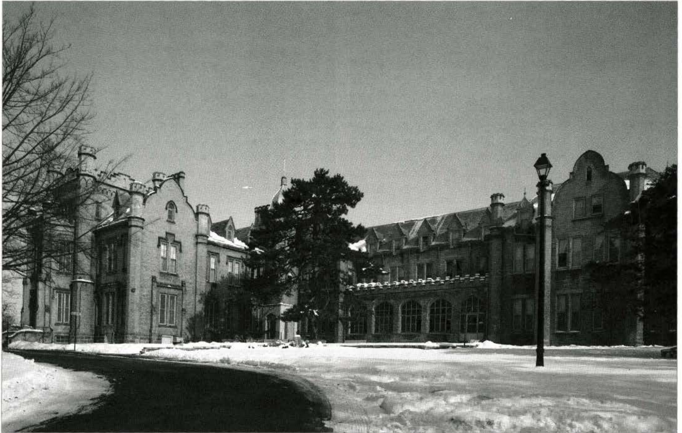
FIG. 10. EXTERIOR VIEW; LEFT: MAIN BUILDING; RIGHT: RYERSON HALL ADDITION. | PHOTO: MALCOLM THURLBY.
