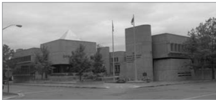
FIG. 32. BRANTFORD CITY HALL, BRANTFORD, ONTARIO; BUILT 1969-1970; MICHAEL KOPSA, ARCHITECTS. | A. WALDRON, PARKS CANADA, 2005.
