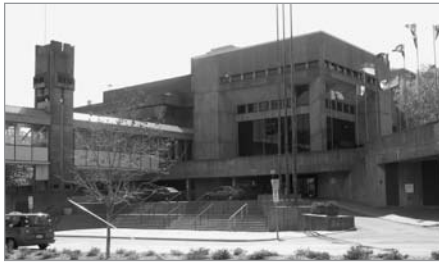
FIG. 31. SAINT JOHN'S CITY HALL, ST. JOHN'S, NEWFOUNDLAND AND LABRADOR; BUILT 1969-1970; JOHN C. PARKIN ASSOCIATES, ARCHITECTS. | A. WALDRON, PARKS CANADA, 2005.
