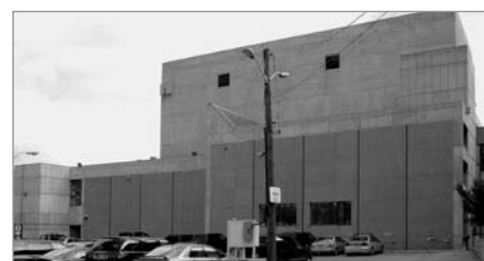
FIG. 15. WEST FAÇADE AND THE PARKING LOT WHERE THE BALLET SCHOOL WAS INTENDED TO BE BUILT. | A. WALDRON, PARKS CANADA, 2007.
