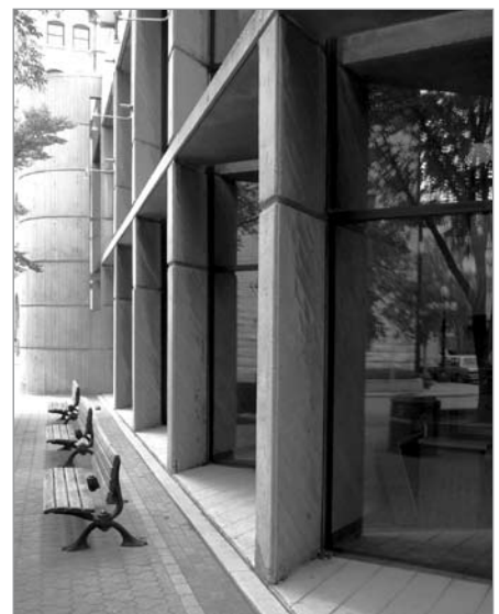
FIG. 11. REINFORCED CONCRETE FORMWORK ON THE EAST SIDE. | A. WALDRON, PARKS CANADA, 2007.
