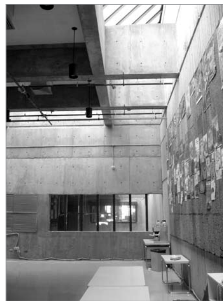
FIG. 25. THE ACTORS' REHEARSAL SPACE WITH THE LIGHTWELL ABOVE AND WINDOWS ACROSS TO THE ADMINISTRATIVE OFFICES. | A. WALDRON, PARKS CANADA, 2007.
