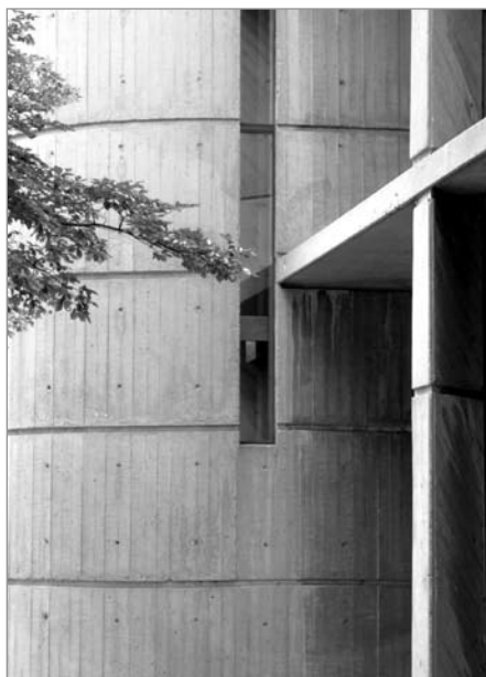
FIG. 12. FORMWORK DETAILING. | A. WALDRON, PARKS CANADA, 2007.
