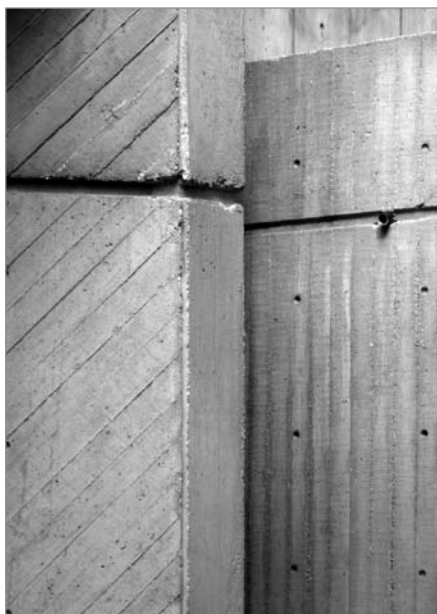
FIG. 13. FORMWORK DETAILING. | A. WALDRON, PARKS CANADA, 2007.
