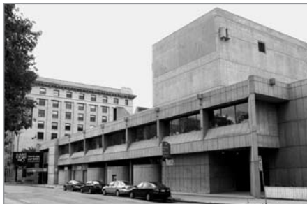
FIG. 5. VIEW OF MARKET AVENUE (NORTH FAÇADE). | A. WALDRON, PARKS CANADA, 2007.
