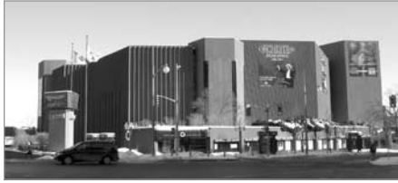
FIG. 30. NATIONAL ARTS CENTRE, OTTAWA, ONTARIO; BUILT 1964-1969; ARCOP, FRED LEBENSOLD, PROJECT ARCHITECT. | A. WALDRON, PARKS CANADA, 2004.
