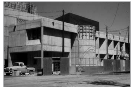
FIG. 10. EAST SIDE OF THE BUILDING DURING CONSTRUCTION. | MANITOBA THEATRE CENTRE, 1970.
