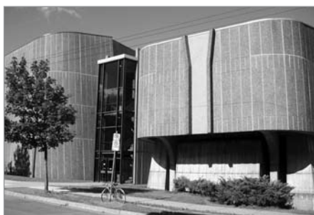
FIG. 34. DALHOUSIE ART CENTRE, HALIFAX, NOVA SCOTIA; BUILT 1969-1971; FOWLER AND ASSOCIATES, ARCHITECT. | WIKIPEDIA.COM, 2007.
