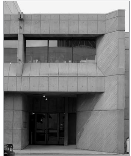
FIG. 6. STAFF ENTRANCE TO THE THEATRE (NORTH FAÇADE). | A. WALDRON, PARKS CANADA, 2007.
