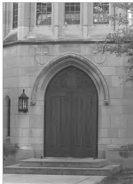
FIG. 5. DOORWAY WITH HOOD-MOULDING, SOUTH DINING HALL, NOTRE DAME UNIVERSITY, SOUTH BEND, IN. | CAMERON MACDONELL
