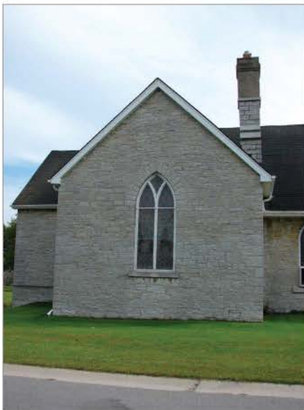
FIG. 35. ST. JOHN'S, PORTSMOUTH, ADDITION OF 1863-1864, FROM THE NORTH. | PAUL CHRISTIANSON, 2011.
