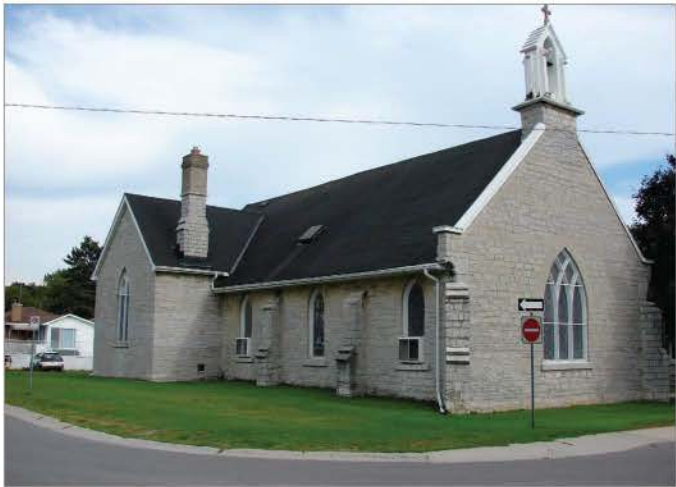
FIG. 34. ST. JOHN'S ANGLICAN CHURCH, PORTSMOUTH, WITH ADDITION BUILT BY JOHN POWER IN 1863-1864, FROM THE NORTHWEST. | PAUL CHRISTIANSON, 2011.
