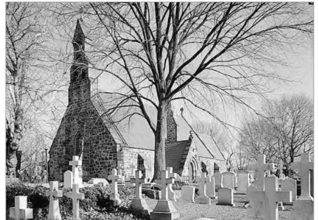
FIG. 4. ST. JAMES THE LESS EPISCOPAL CHURCH (1846-1847), PHILADELPHIA (PA). | [HTTP://WWW.LDC.GOV/PICTURES/COLLECTION/HH/ITEM/PA1153.PHOTOS.137987/PRESOURCE].
