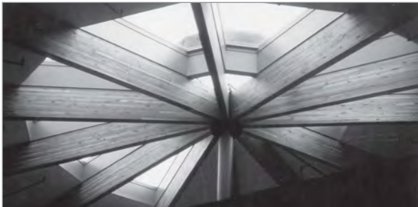
FIG. 8. DOUGLAS CARDINAL ARCHITECT INC. ROSSIGNOL ELEMENTARY. SKYLIGHT. 1973. PHOTOGRAPHER UNKNOWN. | DOUGLAS CARDINAL ARCHITECT INC.
