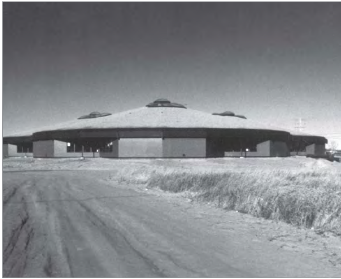
FIG. 10. DOUGLAS CARDINAL ARCHITECT INC. ROSSIGNOL ELEMENTARY. 1973. PHOTOGRAPHER UNKNOWN. | DOUGLAS CARDINAL ARCHITECT INC.
