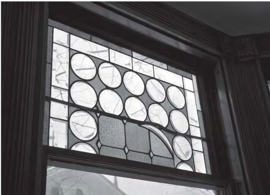
FIG. 1. STAIR LANDING WINDOW AT 96 SECRETARY LANE, 1897. | JOHN LEROUX
