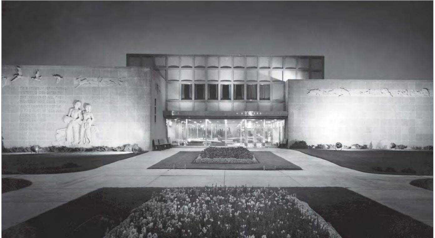
FIG. 10. SASKATCHEWAN MUSEUM OF NATURAL HISTORY (NOW KNOWN AS ROYAL SASKATCHEWAN MUSEUM), REGINA, 1955, E.J. MCCUDDEN, PROVINCIAL ARCHITECT. | HENRY KALEN, COURTESY OF MGM PATTERSON ARCHITECTS.
