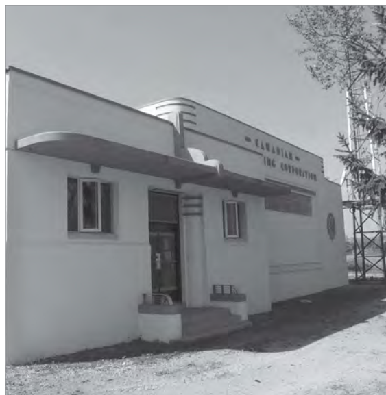
FIG. 4. HORNBY (ON), TRANSMITTER BUILDING, 1937. | MICHAEL WINDOVER.
