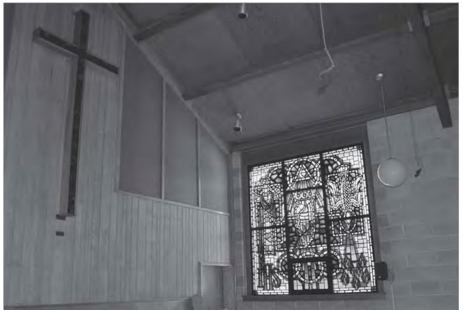
FIG. 18. NASHWAAKSIS UNITED CHURCH CHANCEL WINDOW, P&B STAINED GLASS STUDIO, 1972. | JOHN LEROUX.
