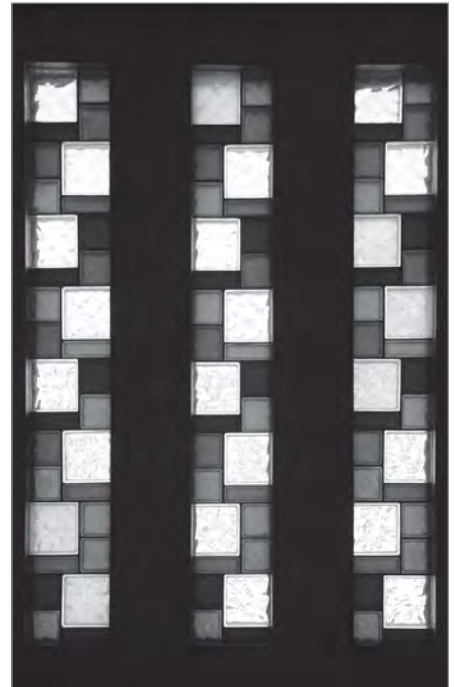
FIG. 5. SALVATION ARMY CHAPEL GLASS BLOCK WINDOWS, NEIL STEWART, ARCHITECT, 1964. | JOHN LEROUX.
