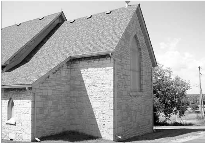
FIG. 33. ST. MARK'S, DETAIL OF THE ORGAN CHAMBER AND CHANCEL ADDED IN 1897. | PAUL CHRISTIANSON, 2006.
