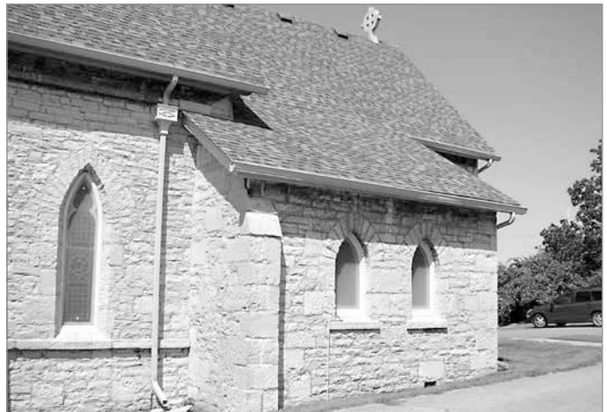
FIG. 32. ST. MARK'S, DETAIL OF LANCETS IN THE NAVE AND THE ORGAN CHAMBER ADDED IN 1897. | PAUL CHRISTIANSON, 2013.
