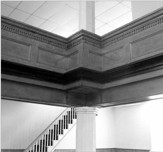
FIG. 9. DESABLE CHURCH OF SCOTLAND, PEI, GALLERY DENTILATION AND BOX FOR CHIMNEY. | JACK C. WHYTOCK.
