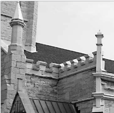
FIG. 22. ST. JAMES' DETAIL OF PINNACLES AND BATTLEMENTS ON ADDITIONS OF 1888-1889. | PAUL CHRISTIANSON, 2013.
