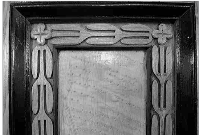
FIG. 6. DESABLE CHURCH OF SCOTLAND, PEI, CARVING DETAIL ON FRONT OF HIGH PULPIT. | JACK C. WHYTOCK.
