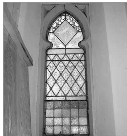
FIG. 19. ST. JAMES' DETAIL OF WINDOW FROM THE SIDE ENTRANCE PORCH. | PAUL CHRISTIANSON, 2014.
