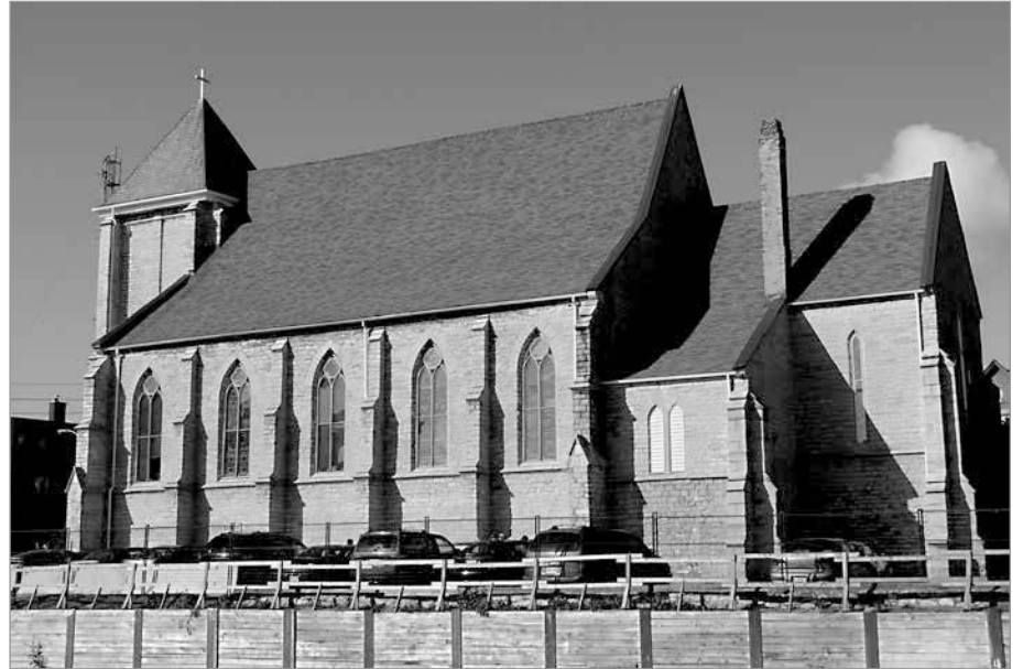
FIG. 5. ST. PAUL'S ANGLICAN CHURCH, FROM THE SOUTH; NOTE THE CHANCEL ADDED IN 1855 AND THE ORGAN CHAMBER PROBABLY ADDED IN 1878. | PAUL CHRISTIANSON, 2008.
