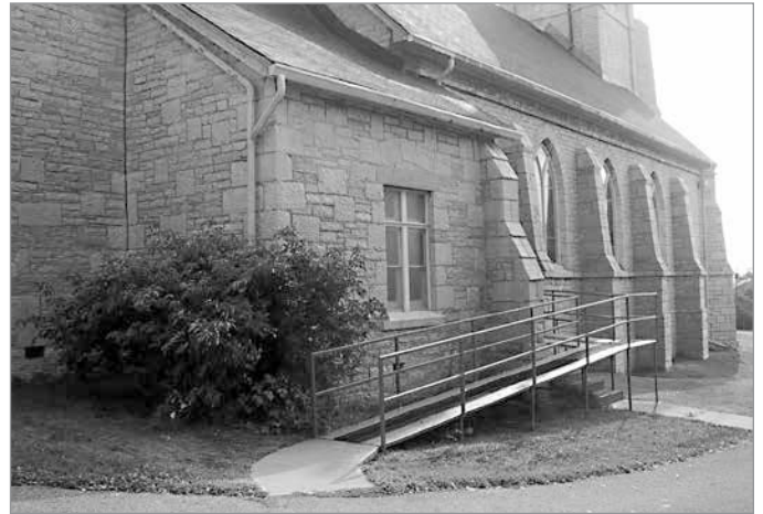
FIG. 34. ST. MARK'S, DETAIL OF NEW VESTRY ADDED IN 1897. | PAUL CHRISTIANSON, 2006.
