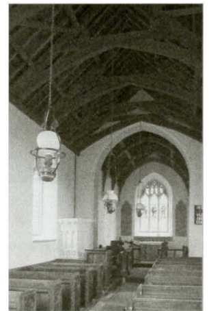
FIG. 16. OLDRIDGE CHAPEL, INTERIOR TO EAST-NORTHEAST FROM NAVE.
