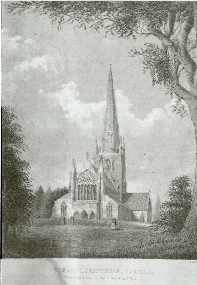
FIG. 2. ST. MARY, SNETTISHAM, NORFOLK, EXTERIOR FROM SOUTHEAST, FRANK WILLS.
