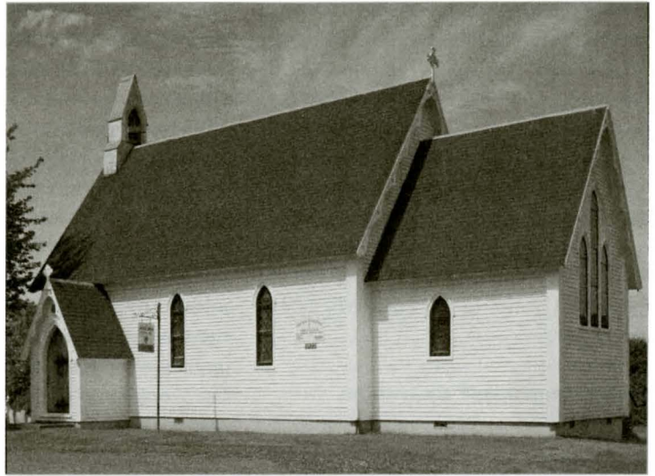
FIG. 47. CHRIST CHURCH, LOWER WOODSTOCK, EXTERIOR FROM SOUTH.
