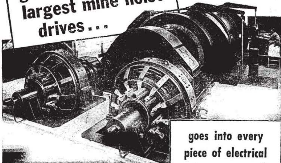
A 4,500/9,000 hp motor-driven hoist at a Northern Ontario mine which is designed to handle over 400 tons of ore an hour from a depth of over 4,000 feet.
