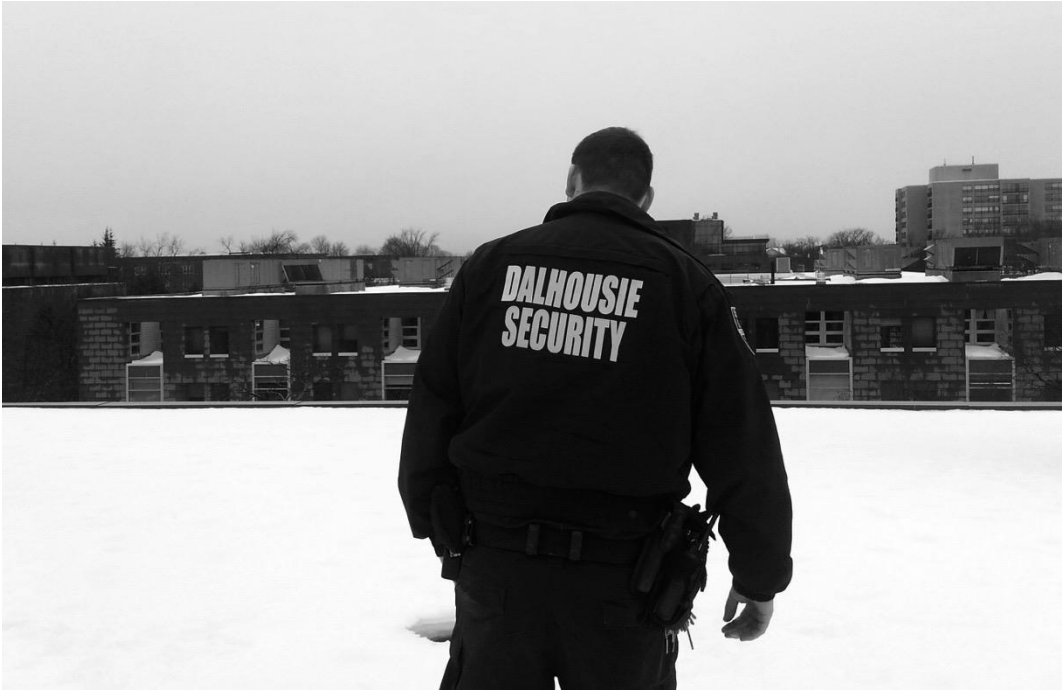
Appendix I6: Officer conducting roof inspection
