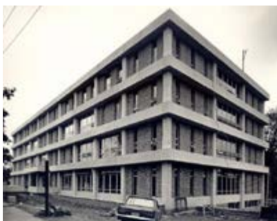
SUB - Under Construction, August 1968
