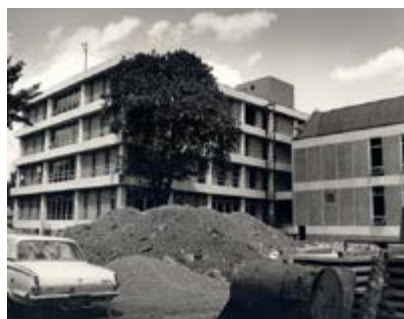
Dalhousie Student Union Building - Construction Shot, 1968
