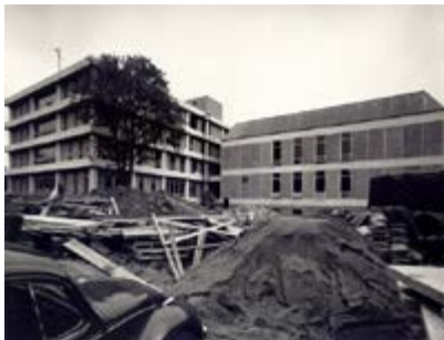
SUB - Under Construction, May 1968
