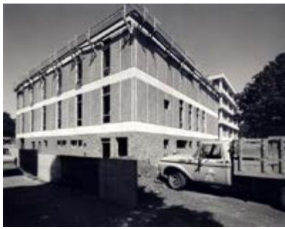
SUB - Construction Shot - June 1968
