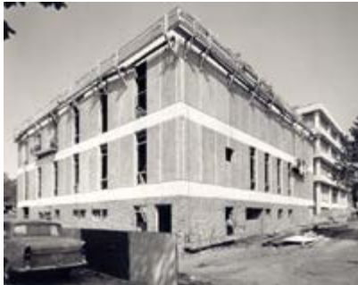
Student Union Building - Construction Shot, May 29, 1968
