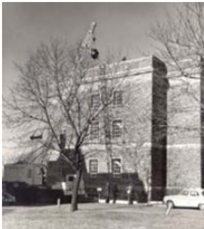
Sir James Dunn Science Building - South Wing, Loading Zone, n.d.
