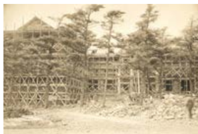
Shirreff Hall Construction, ca. December 1921-December 1922
