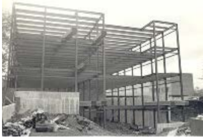
M.M. O'Brien Hall - Construction, n.d.
