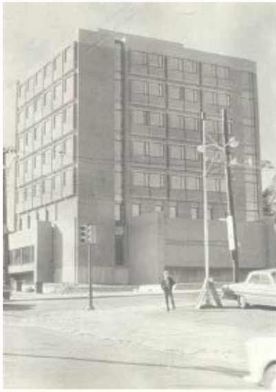
M.M. O'Brien Hall - Construction, n.d.
