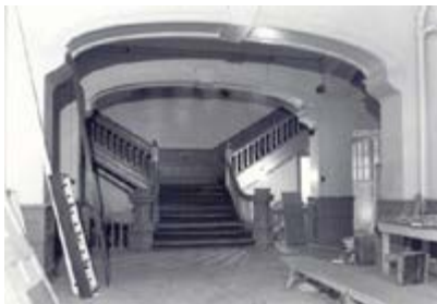
The Forrest Building being restored, 1983
