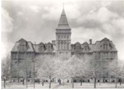
Forrest Building as it was in the 1800s [sic], 1929 (photo dated September 1977)
