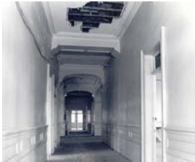
Forrest Building restoration, 1983
