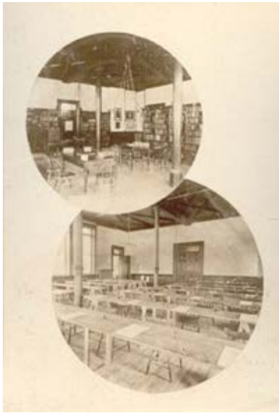
Forrest Building Library and Classroom, 1897
