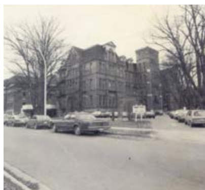
Forrest Building - Street Scene, n.d.
