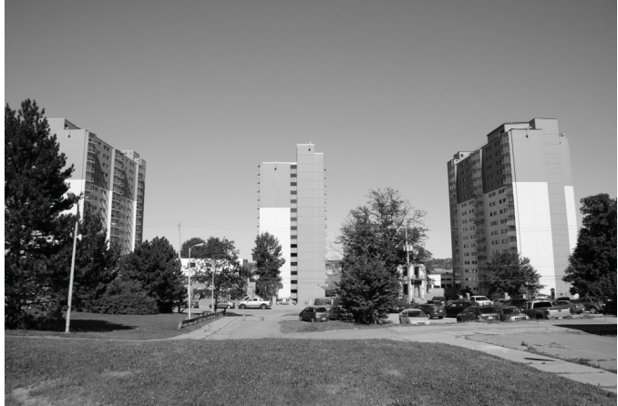
Figure 1.6 View of Harbour View Apartments, looking northeast across Brunswick Street from the site of the school.
