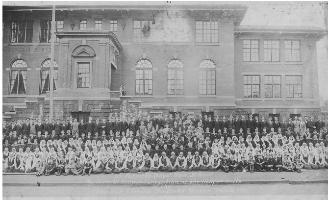
Figure 1.3 The St. Patrick's Boys School, as originally designed by architect Andrew Cobb. (Nova Scotia Public Archives 1931)
