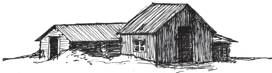
A “half-sod” house, partially sunken into the ground (rear) with a wooden addition (front).
