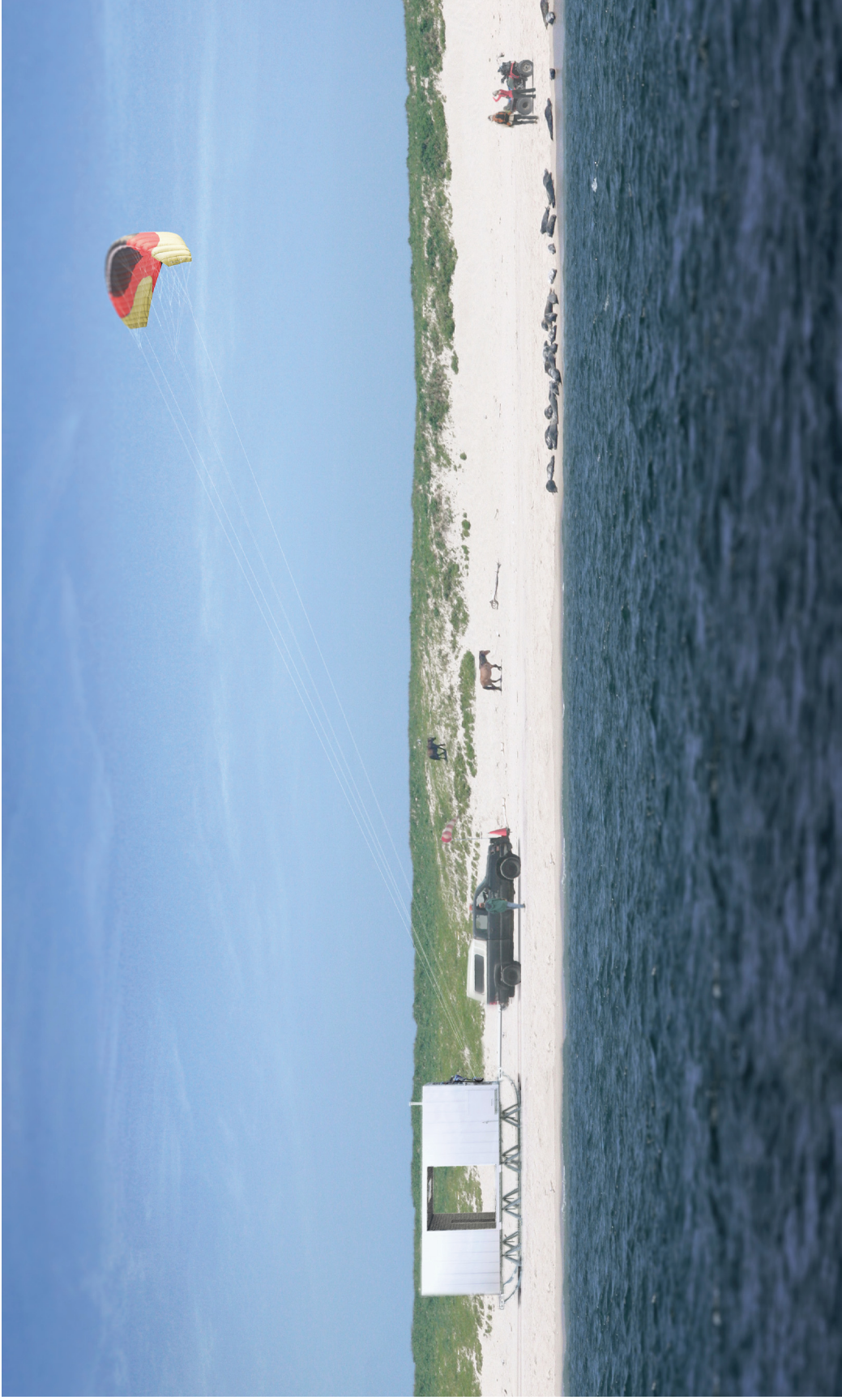
On moving day the shelters can hit the beach to relocate to safer ground. The small island population can easily perform the task with one person to control the kite, one to drive the truck and one to drive ahead to make sure there is a clear path.
