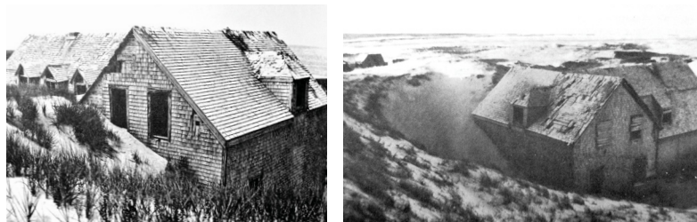
A house being engulfed by sand on Sable Island (Campbell 1974) (left) and (Zinck 1979) (right).
