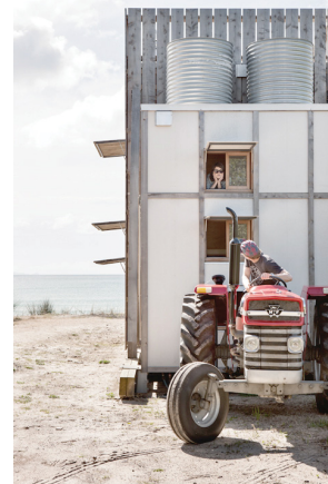
Storm doors / solar awnings being opened (left) (Crosson Clarke Carnachan Architects 2014) Hut being towed by tractor (right) (Crosson Clarke Carnachan Architects 2014)
