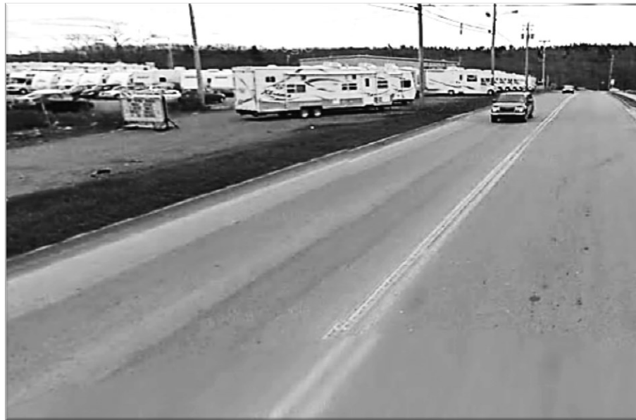
Figure 2-4 Severely rutted road, photo taken at Duke St., Bedford Nova Scotia, October 23 rd 2013.
