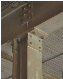
Structural steel connection.
