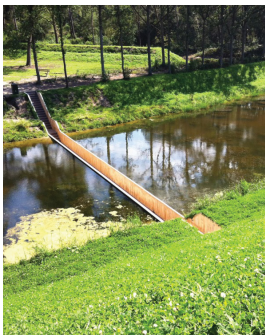
Moses Bridge. (ArchDaily: RO&AD Architecten 2011)
