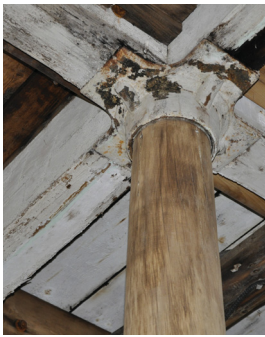
Heavy timber post connection.
