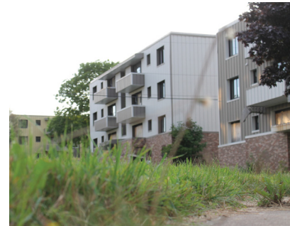
Typical building in Shannon Park
