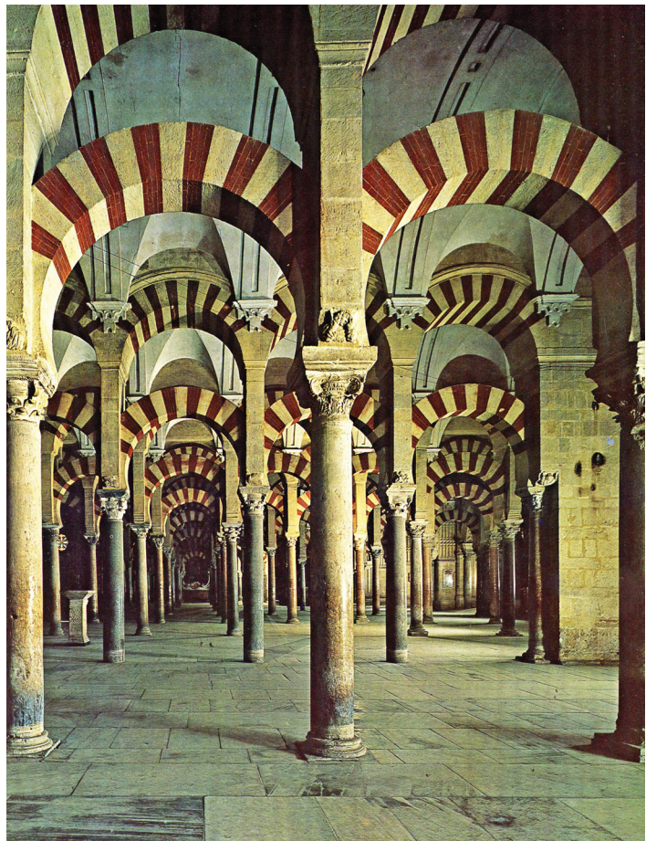
View of arcade in Great Mosque showing reused Roman columns and double arch system, photograph by Fernando Chueca Goitia (Goitia 1971).
