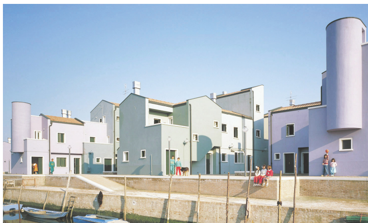
Image of the Housing project in Mazzorbo from the canal. (Veneta 1989, 62)
