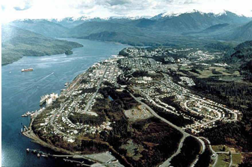
Figure 23. Aerial shot of Prince Rupert that depicts the approximate spill area
