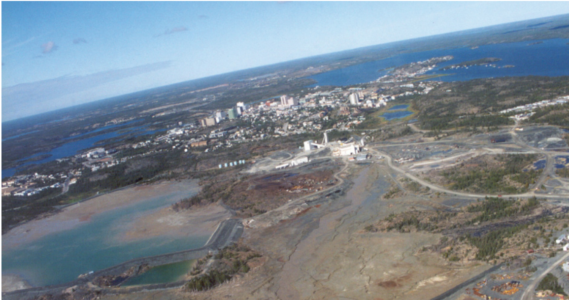
Aerial view of the Con mine property with Yellowknife city centre beyond, 2003 (from Nuna Logistics Ltd, photograph by John Zigarlick)
