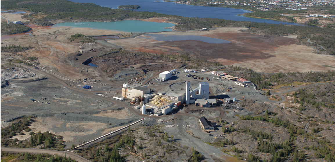
Aerial view of the Con mine's C-1 headframe and processing plant, with tailings ponds beyond (from City of Yellowknife Department of Public Works)
