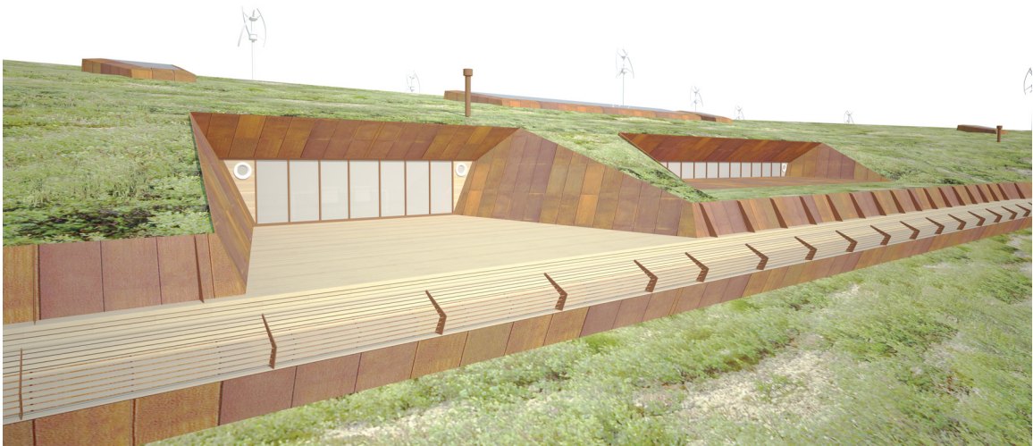
Entry portals accessed from perimeter boardwalk.
