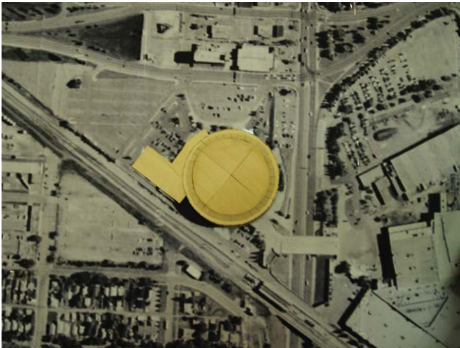
Existing site conditions
