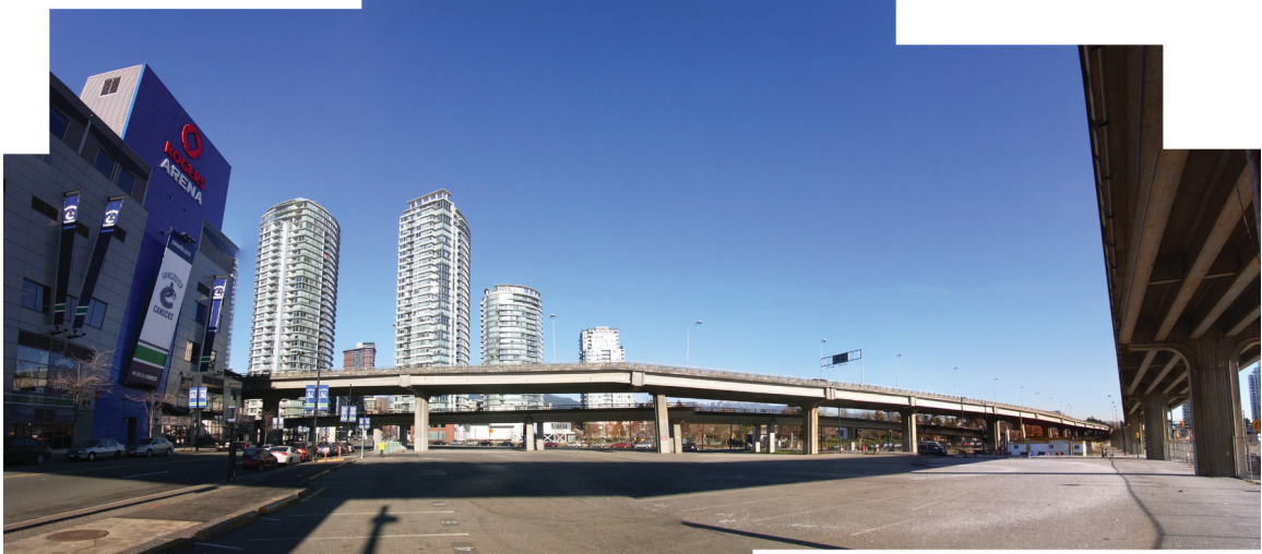
Viaduct building location.
