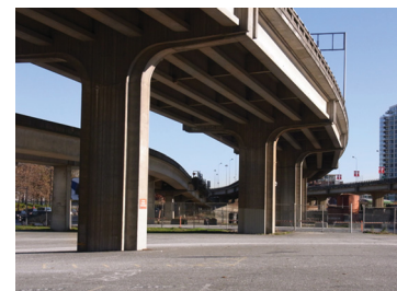
View of Dunsmuir Viaduct from site.
