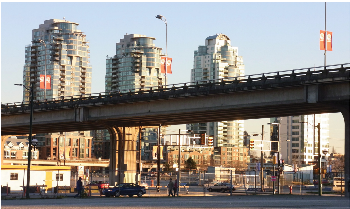
View from viaduct site.
