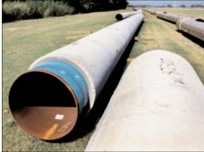
Figure 4.1. Concrete coated pipes, and the uncoated portion. From Ref. [110].
